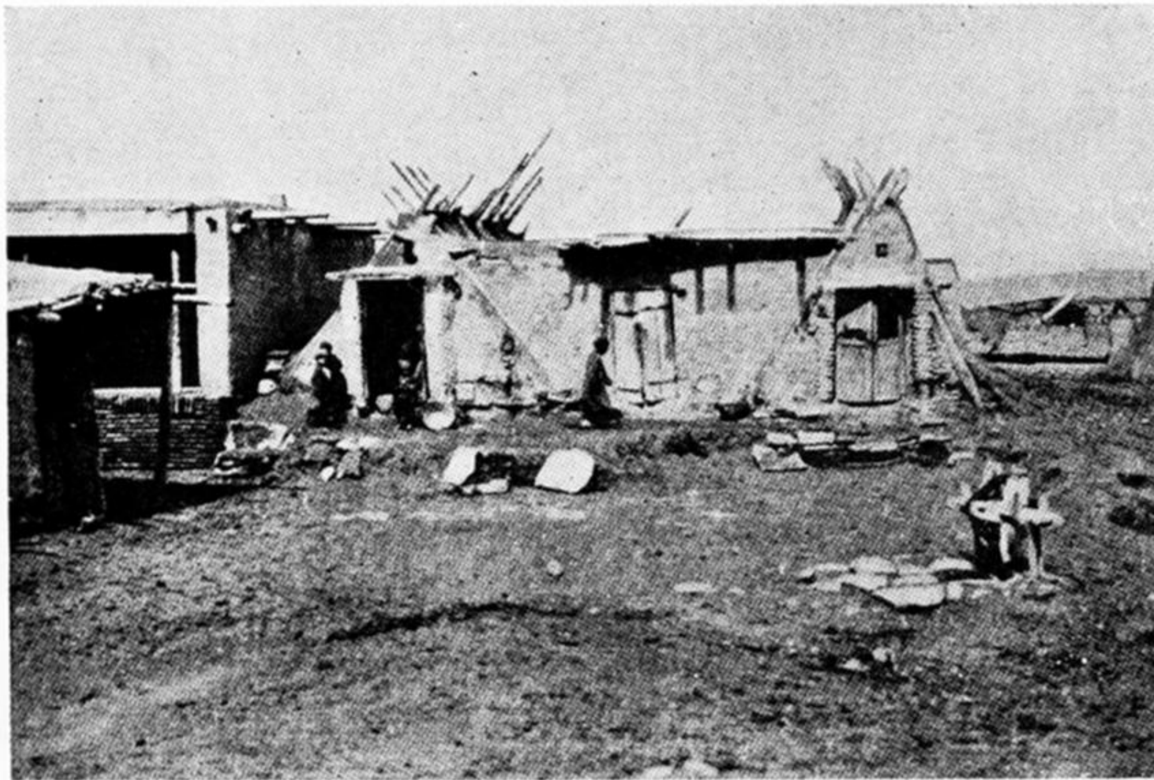
FIGURE 6. Quchan in 1903. After the 1895 earthquake, Quchan was relocated to its present site, but the old town shown in this photograph lingered on. Two 'A' frame shelters built in 1893 or 1895 from roof beams of destroyed houses are seen incorporated into a more permanent dwelling. From Pumpelly (1905, fig. 153).
